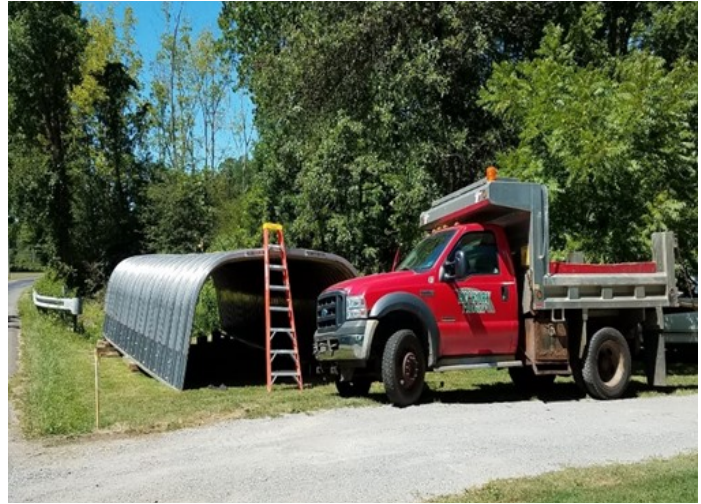
Hickory Township's municipal road crew worked diligently to "build" the arch portion of their new stream crossing in August.
