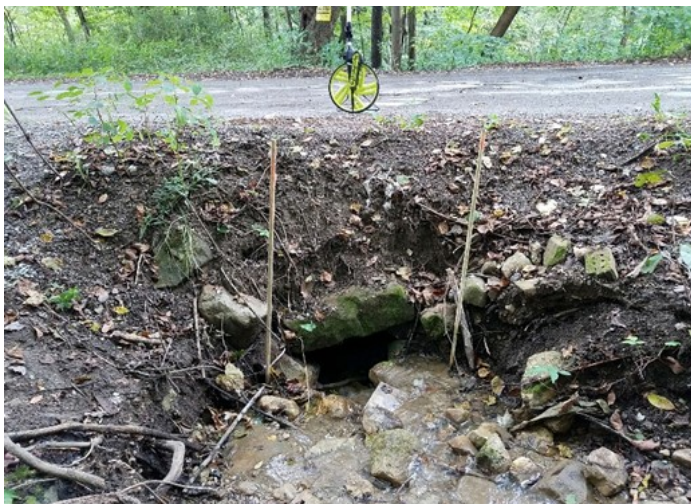
An undersized stream crossing on Evergreen Road in Mahoning Township.
