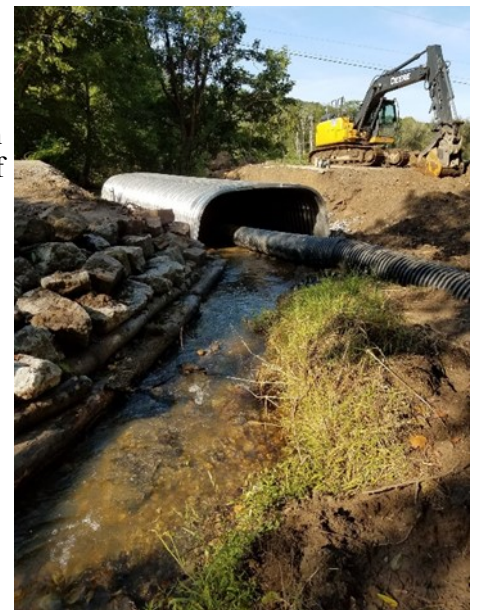
Installation of a bottom less culvert in Hickory Township.
