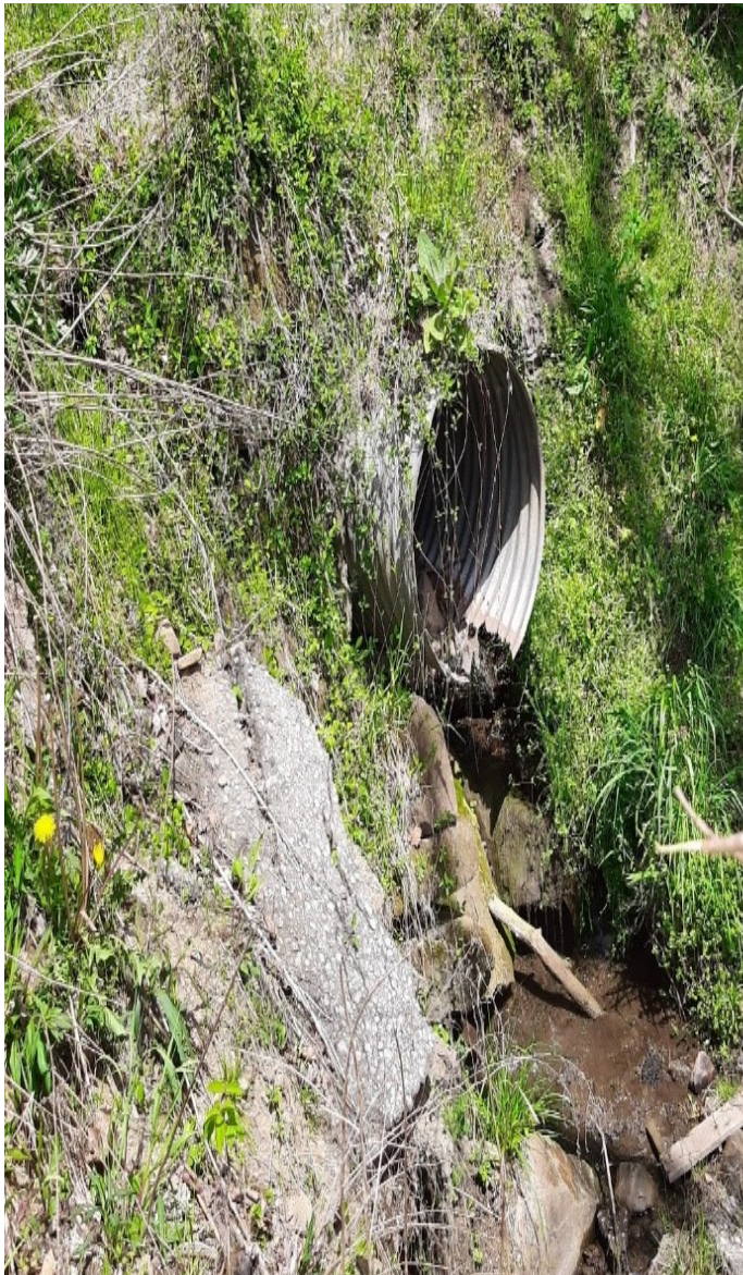
A failing 36-inch cross pipe on Graham Road in Mahoning Township that will hopefully be upgraded during a future DGLVR project.
