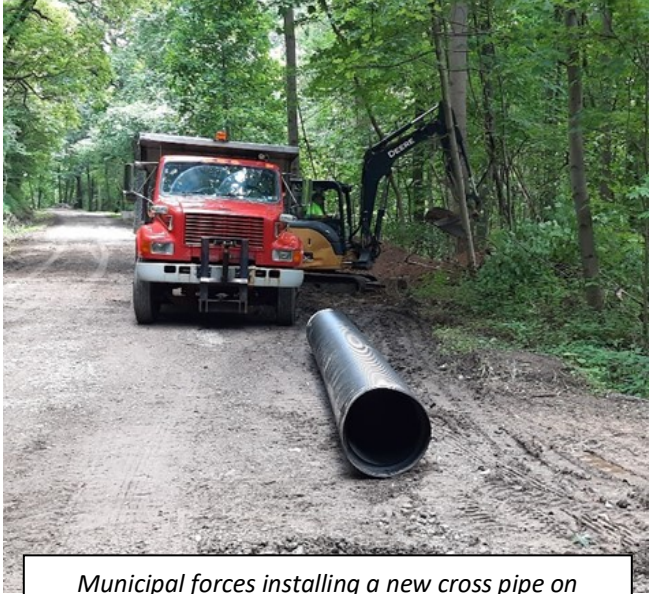
Municipal forces installing a new cross pipe on Chewton West Pittsburg Road.
