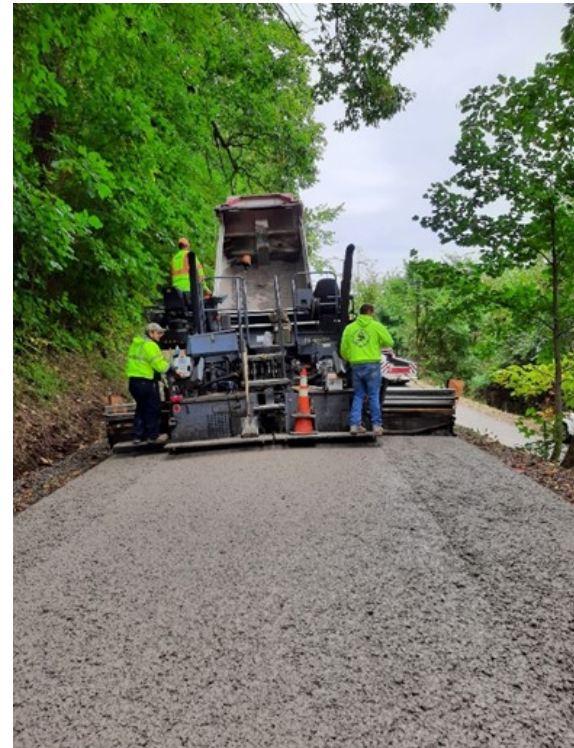
Shenango Township and Youngblood Paving working to place DSA from a quarry in Armstrong Co.
