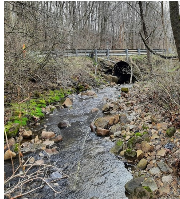
An undersized culvert in Wilmington Township was recently assessed by our staff with help from the Center for Dirt and Gravel Roads.
